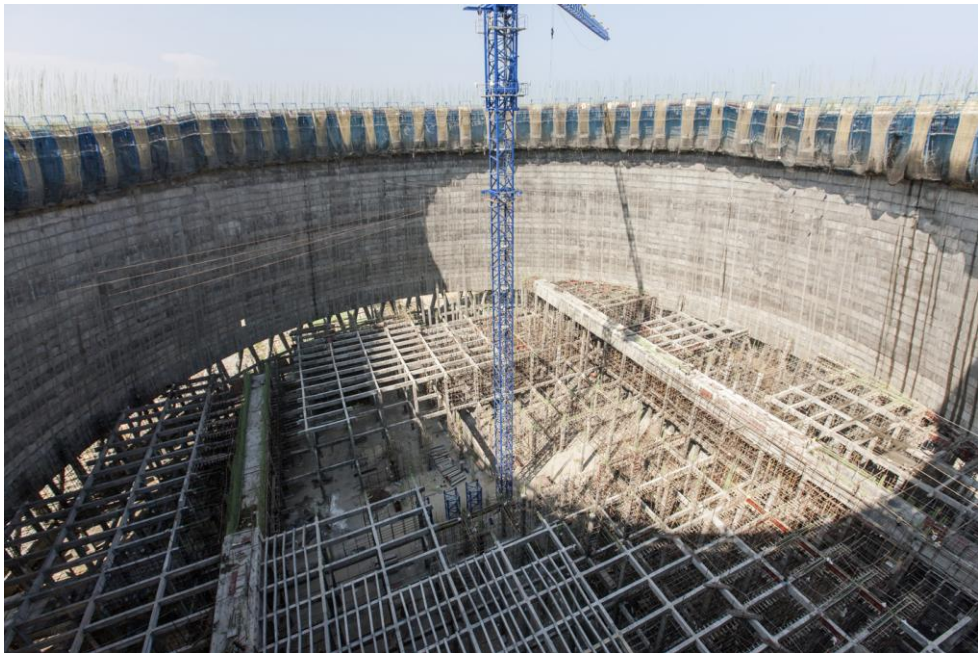
The tower diameter of 132.1 m reduces to 76.4 m at the centre and increases again up to 77.4 m at the top.
