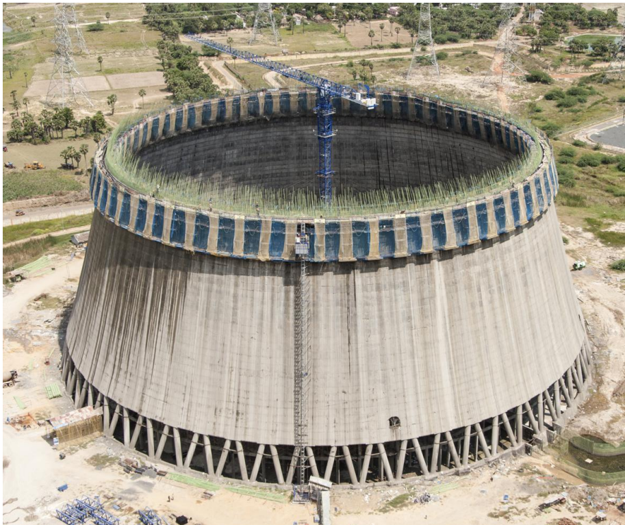
128 self-climbing units of Doka cooling tower formwork SK175 are utilised.
