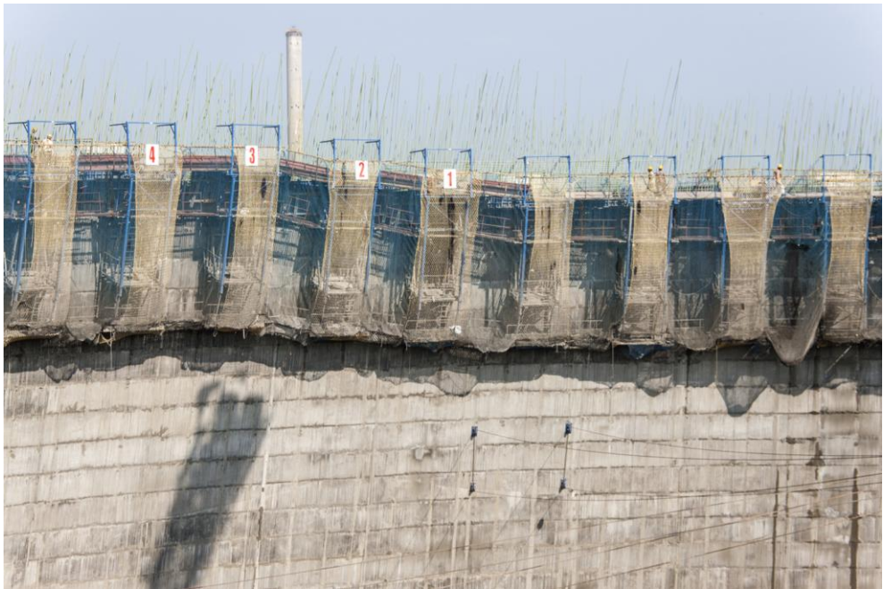
The Doka cooling tower formwork SK175 enables concreting in 1-day cycles.
