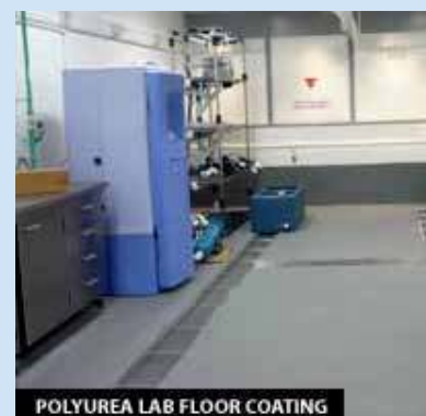
POLYUREA LAB FLOOR COATING
