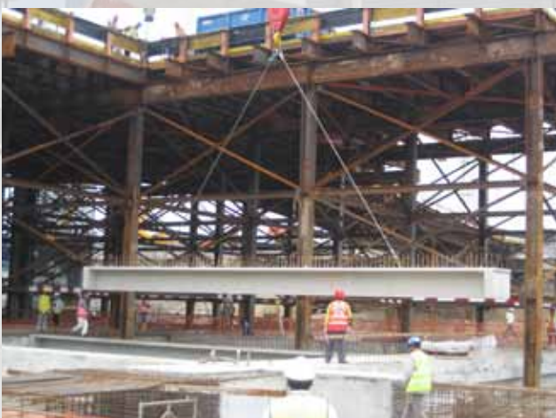
Precast / Prestressed Concrete
