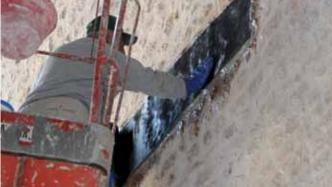
Final phase of laying the MAPEWRAP C UNI-AX fabric.
