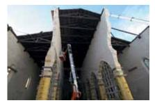
The two main ribs left standing were made safe using a complex network of MAPEWRAP carbon fibre straps.
