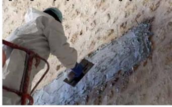
Detail view of laying the MAPEWRAP C UNI-AX unidirectional carbon fibre fabric.
