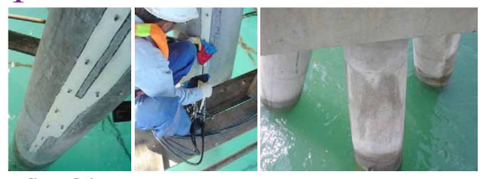
**Signature Park** – Leaking expansion joint in pedestrian underpass. MC-Injekt GL 95 TR TX was proposed. Packer holes were drill at 45° angle towards the joints to intercept the joints. 300mm GEL packers were placed in position followed by material injection. Previous injections using conventional polyurethane had all failed.
