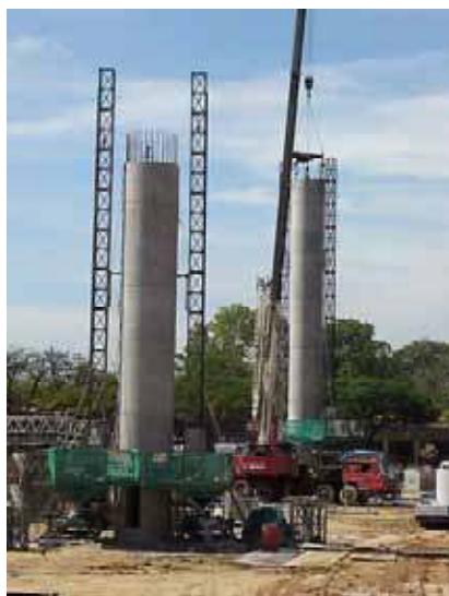
25m Supertree core wall panel installed into position
