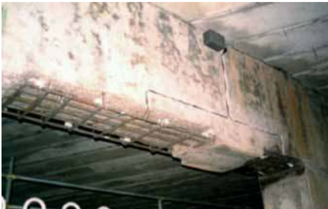
Figure 1 First Monitored Trial of embedded Galvanic Anodes in Patch Repair
