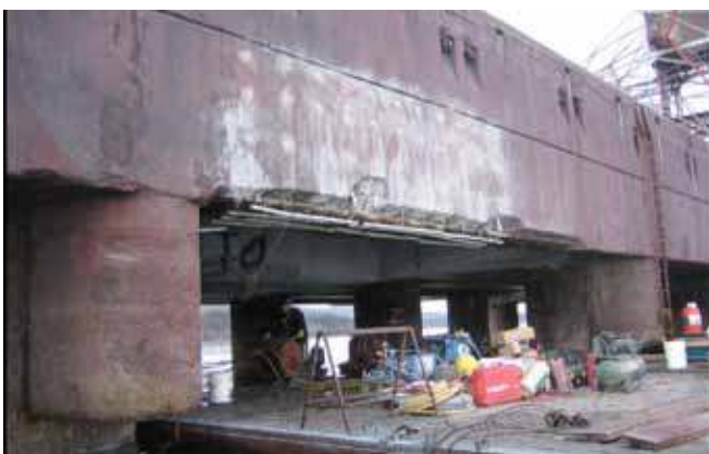
Figure 5 Dilled anodes and line anodes installed at the side and bottom of the girder to control corrosion, Pointe Noire Wharf, Sept-Îles, Quebec, Canada (5)
