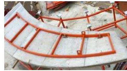
C05 Precast spiral flight permanent formwork panel
