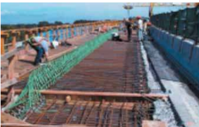
Figure 3 Anodes installed at the edge of existing deck for the deck widening to prevent corrosion from initiating, Port Mann Bridge, Vancouver, British Columbia, Canada
