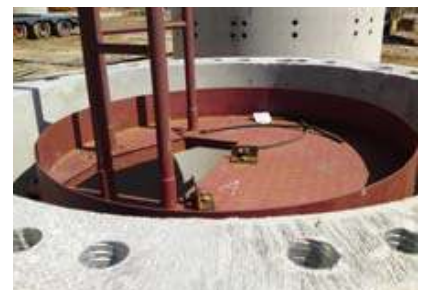
Core wall internal access platform pre-fixed to alternate level of panel before installation enhances work safety
