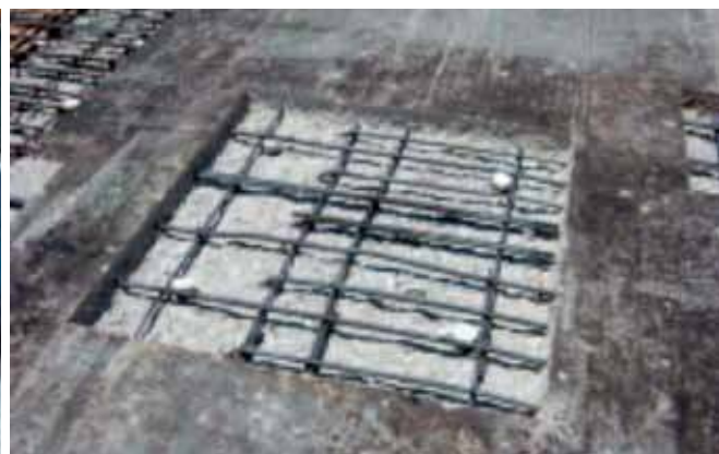
Figure 4 Anodes installed around the perimeter of a bridge deck patch, shallowater, texas, usa
