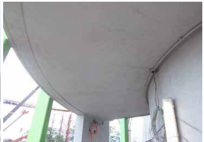
open spiral staircase soffit using precast formwork panel
