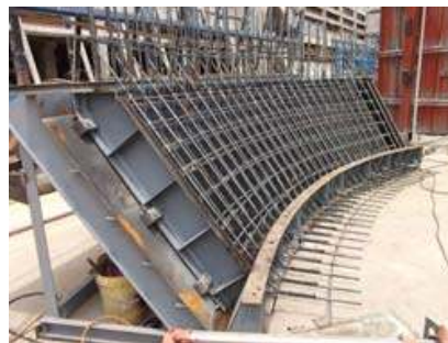
Precasting Back of house inclined wall
