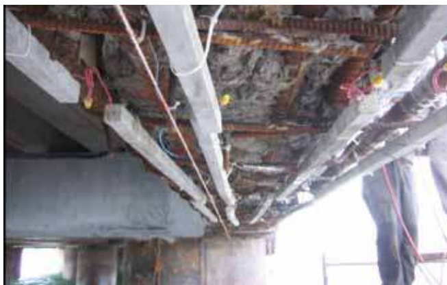
Figure 8 In 2006 Distributed anodes installed at the bottom of the girder to control corrosion, Pointe Noire Wharf, Sept-Îles, Quebec, Canada. Currents from the anodes ranged from 10-20mA/m 2 depending on the seasons, and the polarization was well above 100mV
