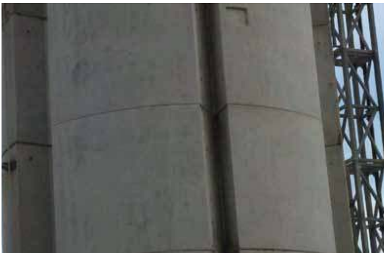
50m C05 installed precast main cores with services compartments
