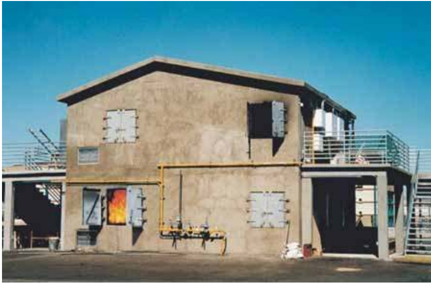
A burn facility in the fire-training industry
