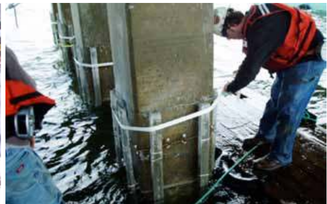
Figure 9 In 2006 DAS anodes installed in concrete jackets for 764 reinforced concrete piers supporting Robert Moses Causes, Long Island, New York, USA. Polarization is well above 100mV and the projected service life is more than the design service life of 35 years
