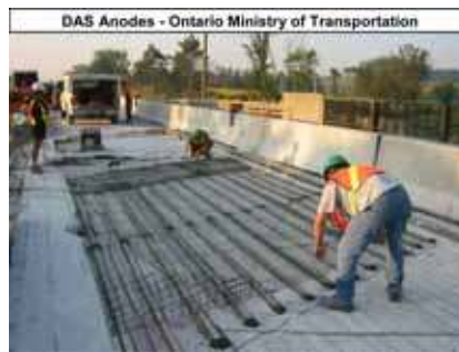
Figure 7 First Trial of DAS anodes in a Bridge Deck Overlay, Ontario, Canada, 2003
