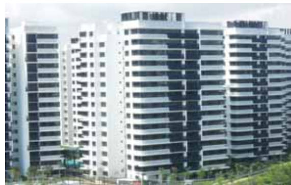
PBU & Precast for N V Residence
