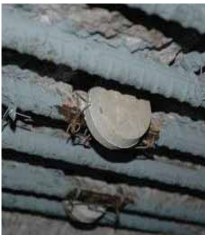
The specification of corrosion repairs using sacrificial anodes for a reinforced concrete tunnel
