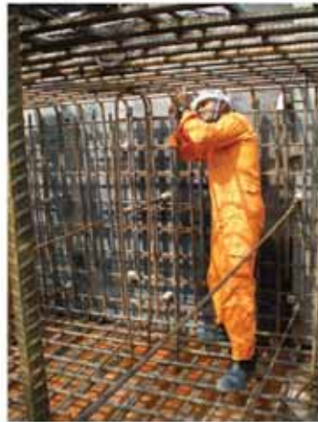
installing temperature monitor
