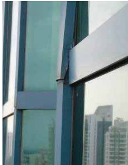
Typical defects noted including the loosening of aluminium finishes
