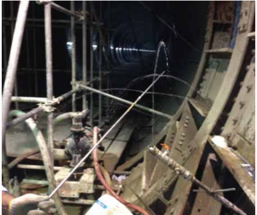
Figure I shows the general layout and concrete were raised of how to stabilise area underneath the existing tunnel segments.
