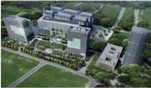
Mapletree Business City at Alexandra
