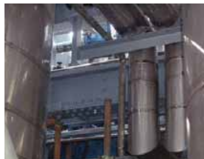
Inspection revealed corrosion treatment and replacement of some I beams required
