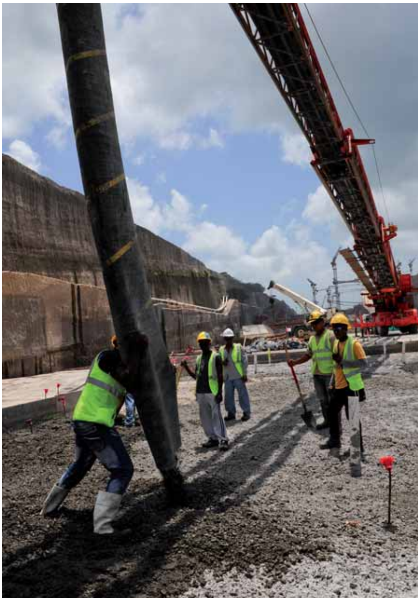
Above. For this building project Mapei developed a new tailor-made admixture: DYNAMON XP2 EVOLUTION 1. The concrete made with it features excellent workability and ease of application.
