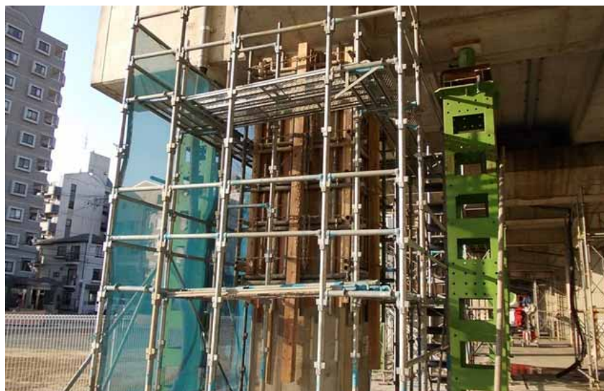
Apparent condition of installation of mold
