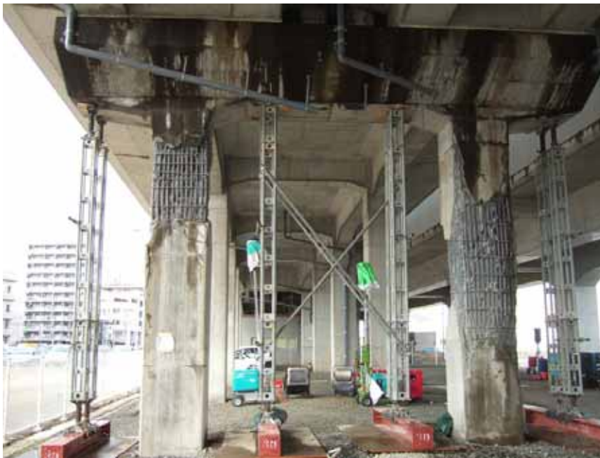
Reconstruction of pier (Tōhoku earthquake and tsunami)
