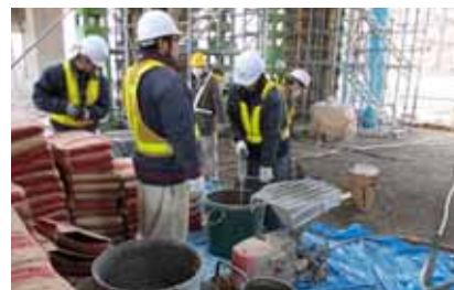
Mixing and injection of quick hardening non shrink grout
