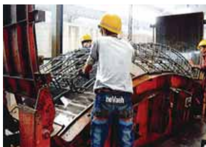
Figure 3. Workers placing rebar cage around mould.
