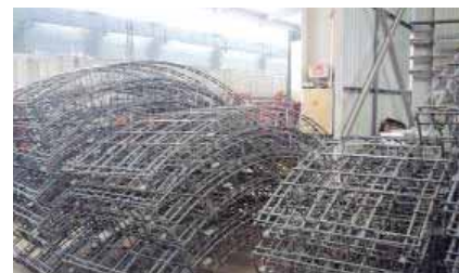
Figure 1. Prefabrication and storage of rebar cages.
