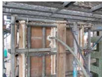
Injection of quick hardening non shrink grout
