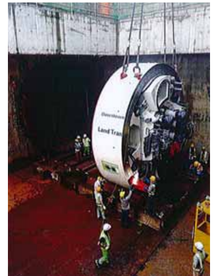
Figure 14. TBM Assembly inside Launch Shaft.
