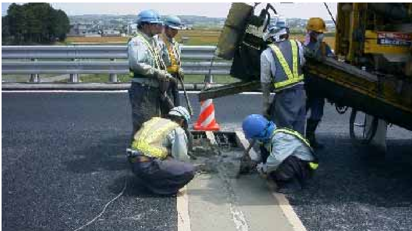
Repairing for the bridge, expansive joint
