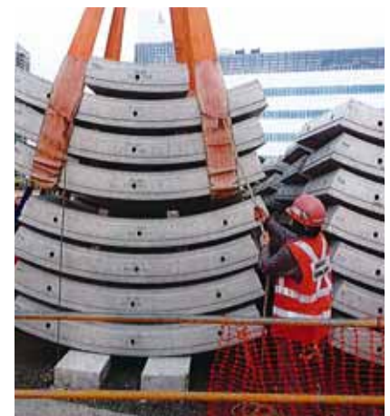
Figure 15. SFRC segment transportation from storage yard to launch shaft.
