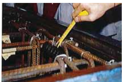
Figure 4. Covers around rebar cage inside segment mould.
