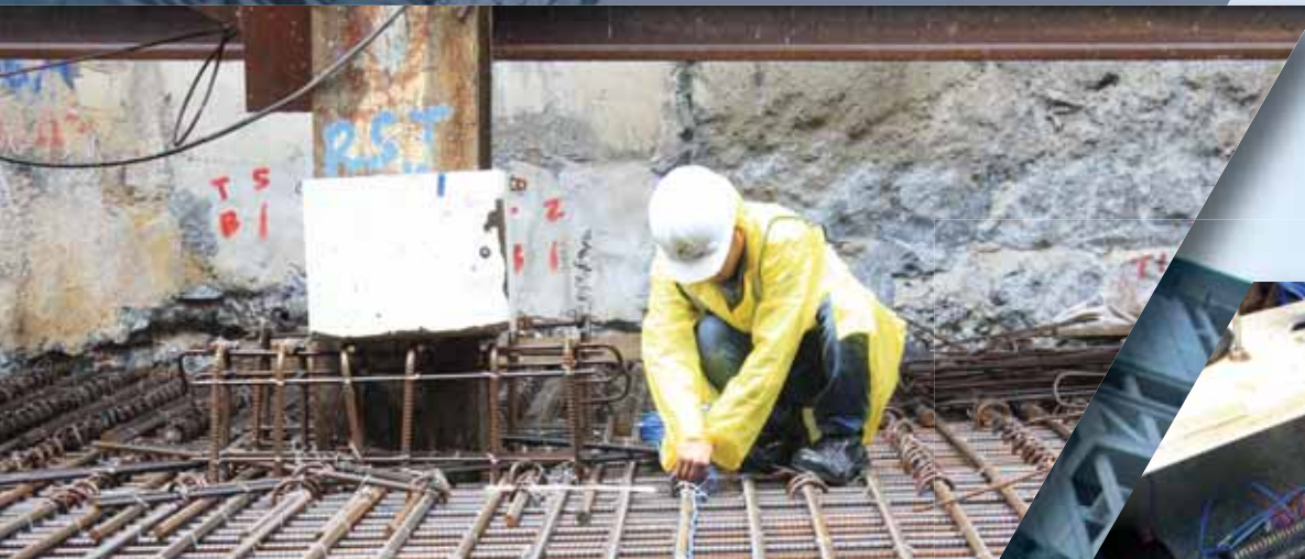
Installing temperature control monitoring system
