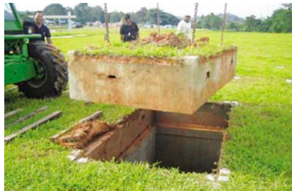
Crypt cover with turf is lifted for burial and easily reinstated. Mechanized lifting frame can be used to break the suction force on the crypt cover
