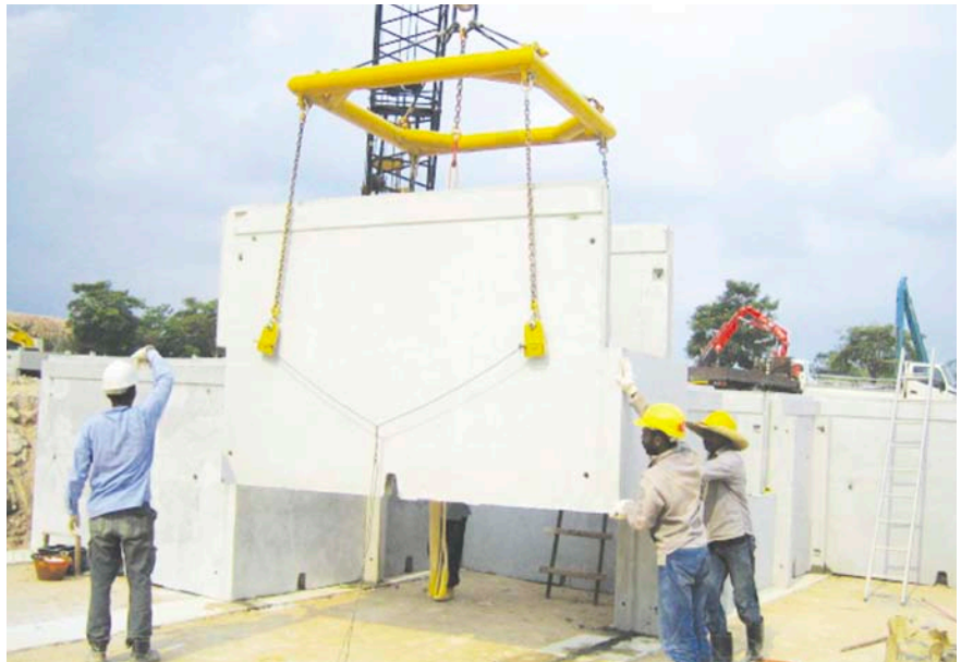
Assembly of crypt components. Arrangement of the crypts is compact, neat and scalable
