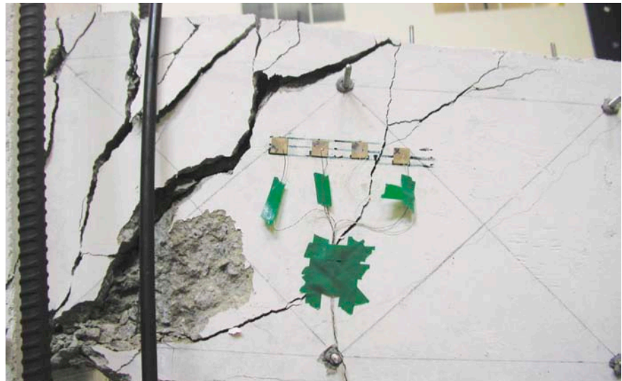
Position of PZT sensors and cracks in specimen
