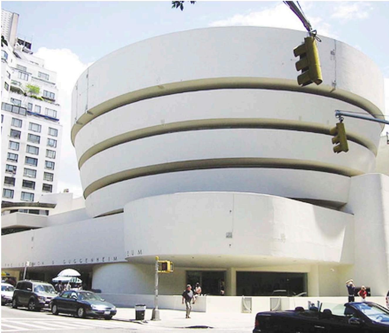
2007-2008: repairing of certain sections of the Museum's circular outside facade using PLANITOPXS mortar.
