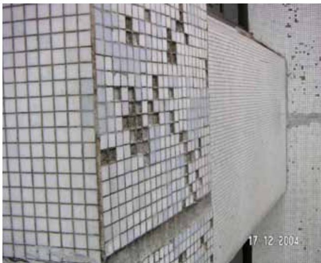
Figure 3 Spalling of mosaic tiles on precast mullion
