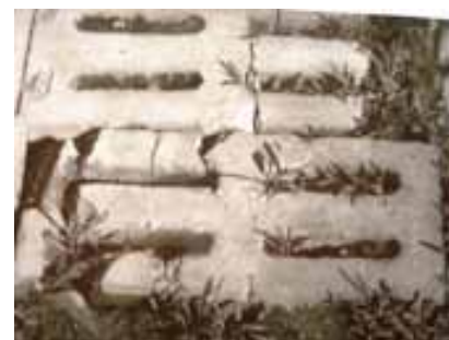
Fig. 2: Cracked reinforced concrete pavers
