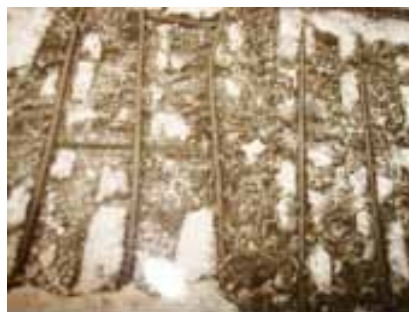
Fig. 1: Deteriorated reinforced concrete pavers
