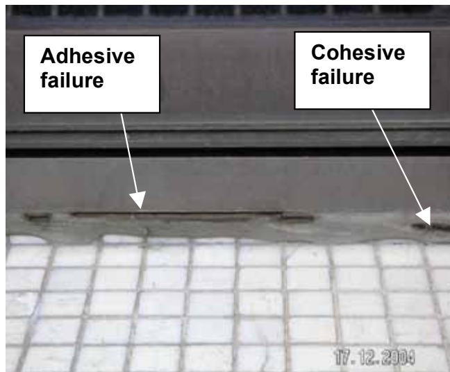
Figure 4 Adhesive and cohesive failure of the sealant
