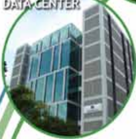
JURONG DATA CENTER
