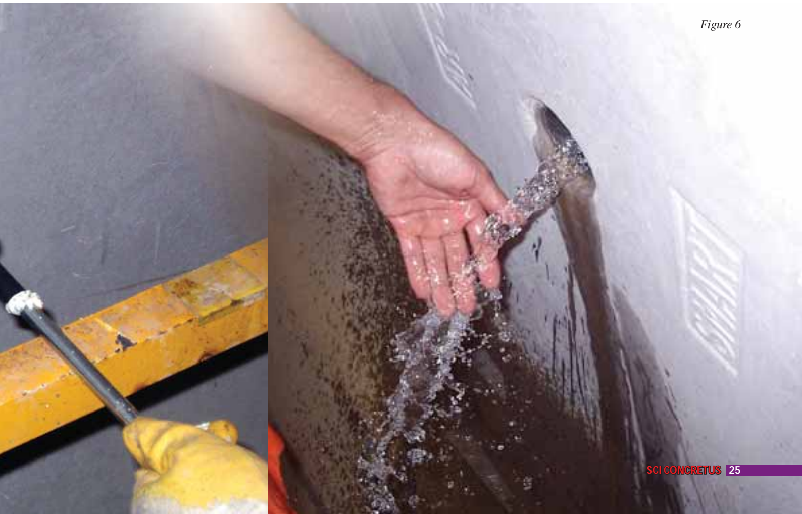
Figure 5. Tunnel joint injection with MC Injekt GL 95 TR TX in SMART Tunnel
