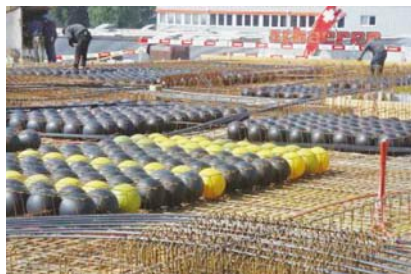
a) Void formers installed in formwork
