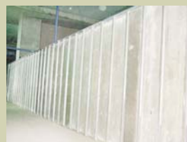
No Lintel (up to 4.3m height) No Stiffener (up to 6m span)
