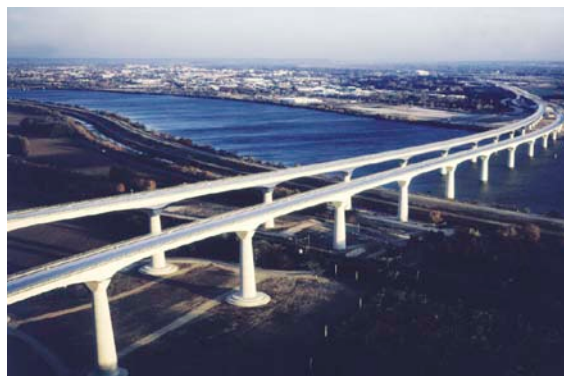
b) Avignon TGV Viaducts, France
