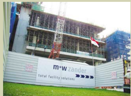
Jurong Data Center
