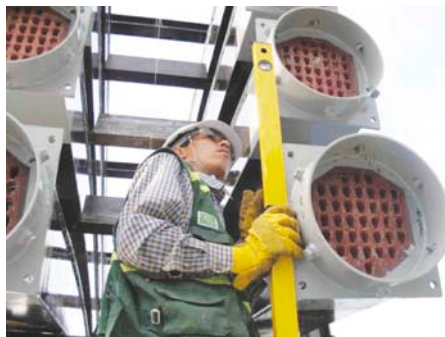
b) Extradosed tendon saddle (VSL system)
