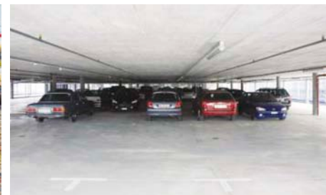
b) Finished floor slab
